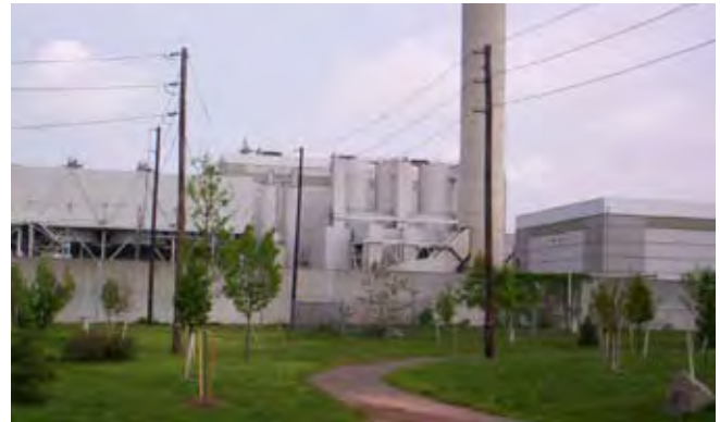
The New Jersey Forest Service replanted trees on residential and commercial property. In the background is an electrical plant where trees removed due to ALB were used to generate electricity.
